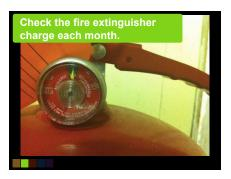
**27:** Ensure the extinguisher is fully charged and ready for use
