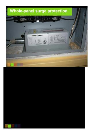
**48:** Install surge and lightning arresters at all electric service panels to buildings to protect interior wiring and electronic equipment.
